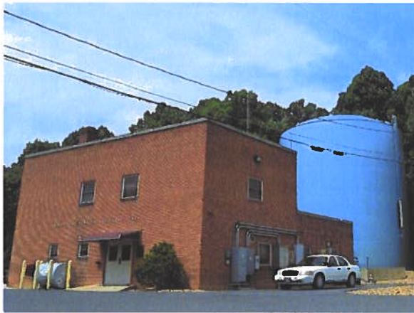
Bridgewater's Water Treatment Plant
