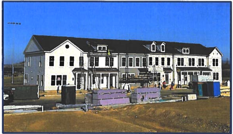
Image 4. Townhomes under construction near Turner Ashby Drive.
