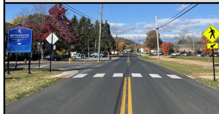
Mt Crawford Avenue Crossing at Naomi Lane.
